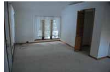
Remodeled Upstairs Bedroom
